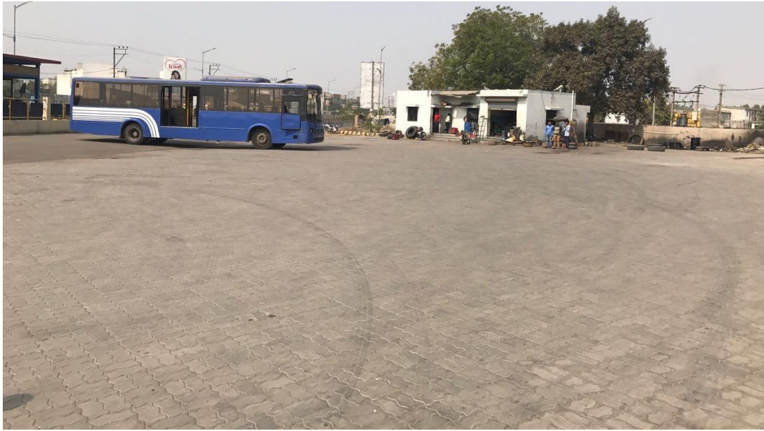
FIGURE 76: BRT DEPOT IN RAJKOT
