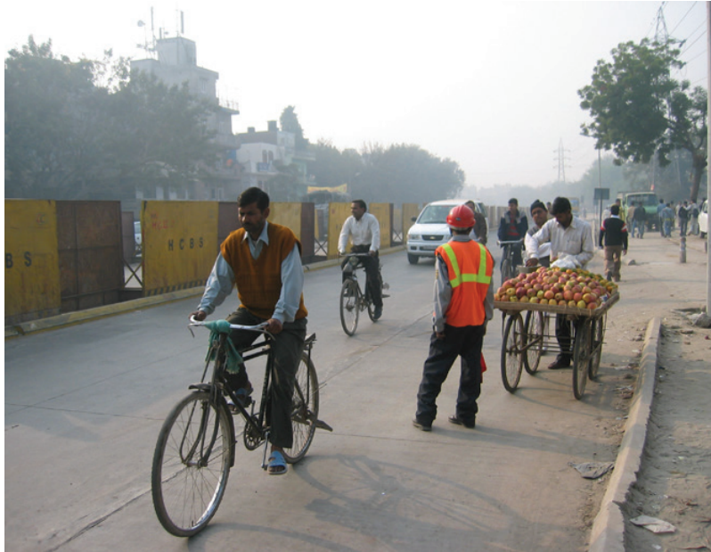
Figure 42 : Cyclists move with other traffic in the traffic control zone during construction. (Source: Delhi)
