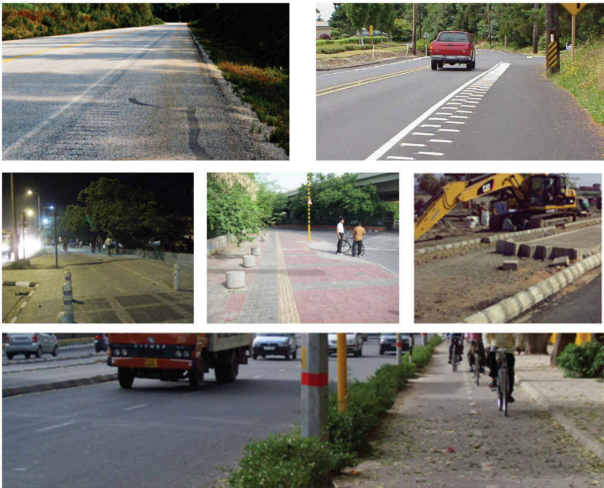
Figure 30 : Edge Treatment : Deterrent Strip (top) www.cyclotouringbc.com/ (L) www.pexco.com (R), Bollards (Middle-L)&(Middle-C), Curb laying at Rajkot BRT (Middle -R)Green & Utility Belt, Delhi BRT (Bottom)
