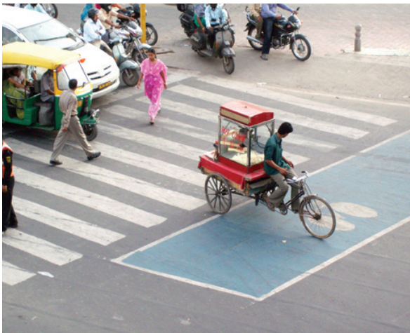
Bicycle box at BRT Corridor, Delhi
