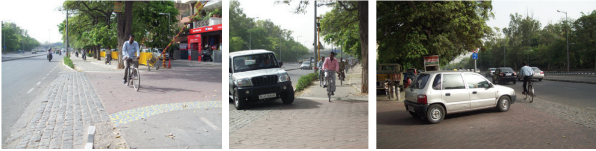
Figure 29 : Traffic Calming measure - Table Top Crossing at Bus Rapid Transit System, Delhi (Source: TRIPP, Delhi)
