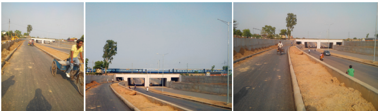
Figure 24: Figure 24: Grade Separated Crossing for NMV (ongoing construction), Chandigarh
