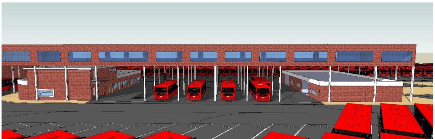
Figure 46: View of bus maintenance facility
