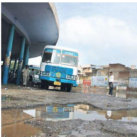
Figure 2: Dilapidated Bus Terminal, Gurgaon (hotgurgoan.com)
