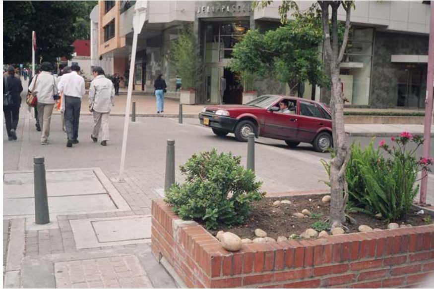
Figure 10: Raised platform treatment for pedestrian paths across entrance/exit to side lanes and service lanes in Bogota, Columbia
