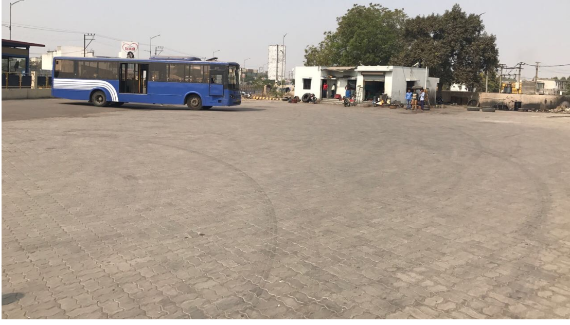
FIGURE 76: BRT DEPOT IN RAJKOT
